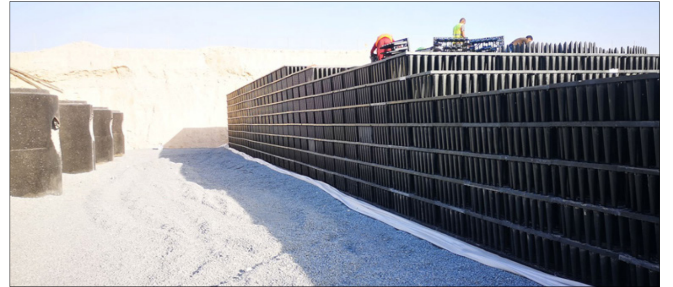
Infrastructure, South Al-Mutlaa (KW)
