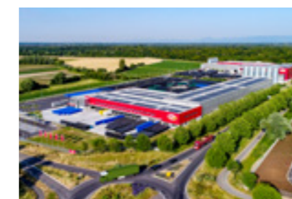
Production site in Neuried (Germany)
