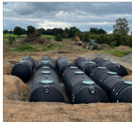
Installation of Installation of 868 PE oneAdvanced, Dundrum House Hotel
