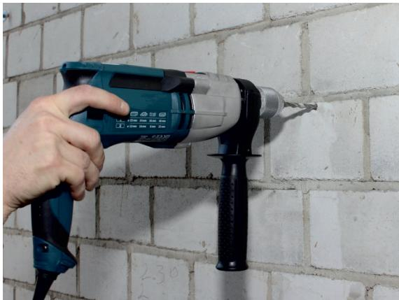
The control must be installed in a dry and dust free interior. Two 8 mm holes must be drilled into the wall for assembly.
