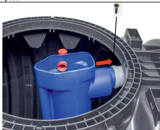
Insert the sampler's outflow connection into the sleeve of the outflow pipe (use lubricant!). The sleeve connection must be secured with a Spax screw.
