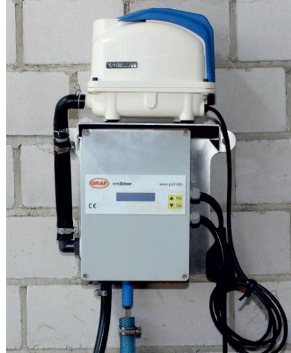
Connect the air hoses to the control's hose nozzles. We recommend heating the hose ends for assembly.
