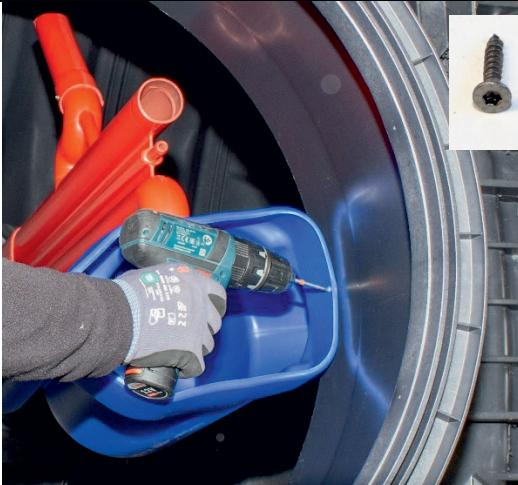
Secure the sampler to the tank dome with a Spax screw.
